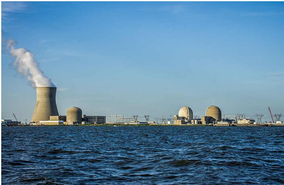
Salem and Hope Creek nuclear reactors
